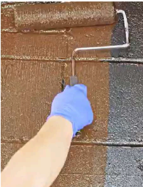
Foundation Sealant dries black
